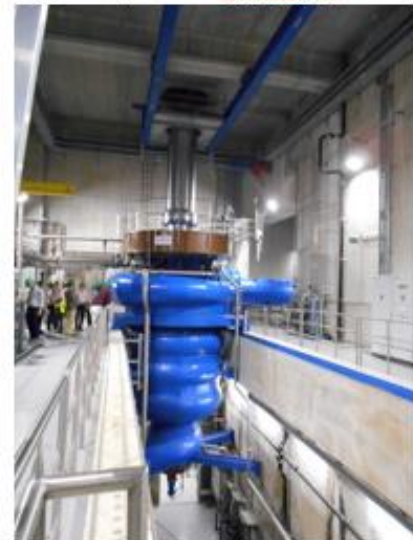
Reverse pump at the Veytaux pump storage installation
